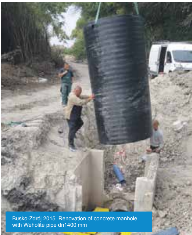
Manhole under renovation
